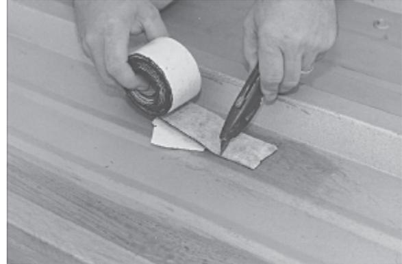
**FIGURE 2.6:** Seal fasteners with Metal Guard Seam Tape and Guardian General Purpose Primer. Lightly prime fastener area before application of tape and then prime surface of tape after application.
