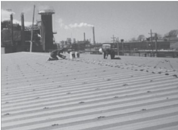
**FIGURE 2.2:** Tighten all fasteners. Replace missing, stripped or damaged fasteners.
