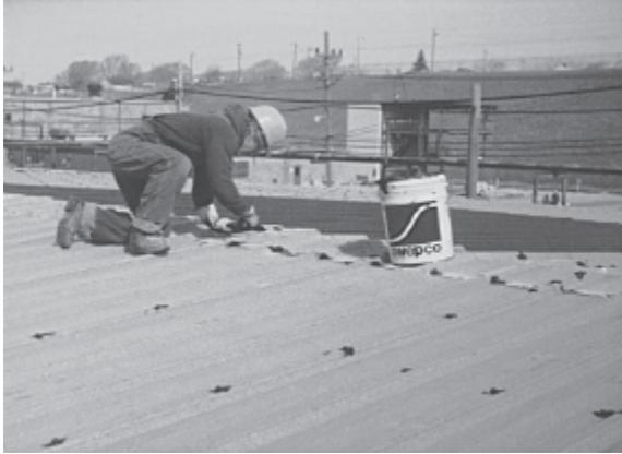
**FIGURE 2.1:** Insure panel tightness and replace any damaged panels.
