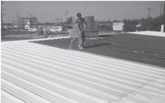
**FIGURE 2.7:** Coat the sealed roof with SWEPCO Aluminum Roof Coating or White Acrylic Coating.
