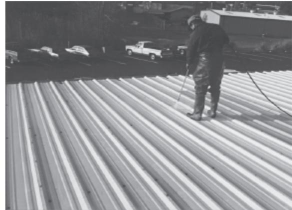
**FIGURE 2.3:** Clean the roof surface thoroughly.
