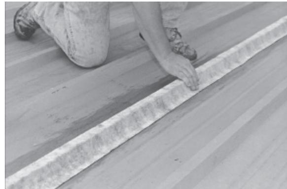
**FIGURE 2.5C:** Rub firmly to remove air pockets and insure complete contact with surface.
