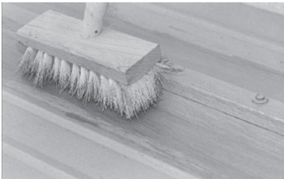
**FIGURE 2.5A:** Lightly prime seams and joints with Guardian General Purpose Primer. Allow to dry until clear.
