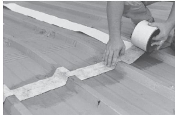
**FIGURE 2.5B:** Seal primed seams and joints with Metal Guard Seam Tape. Remove backing paper and center over primed seam or joint.
